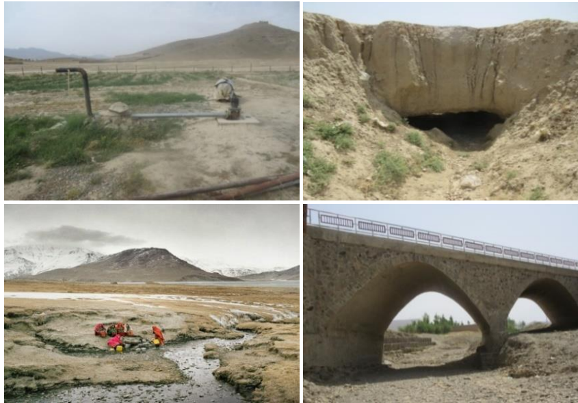
Fig. 2.12 Water problems in Dawlatzai Village Paktya Province
