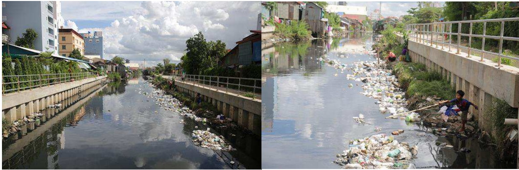
Figure 2-1 Wastewater discharge channel in Phnom Penh
